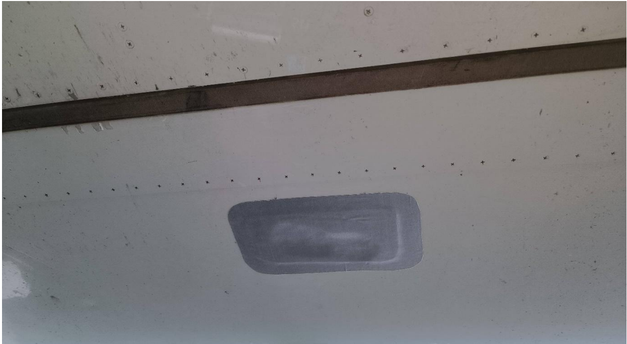
Figure 13. Crack to left hand wing inboard aft flap lower skin covered by speed tape
