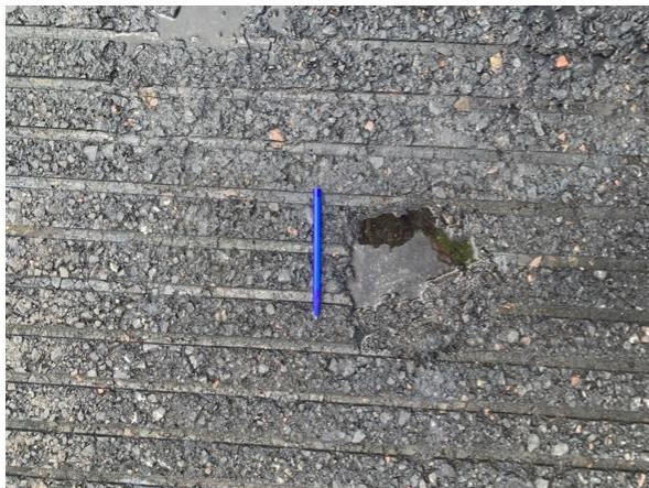
Figure 3: Crater created on the runway where the left main gear came to rest
