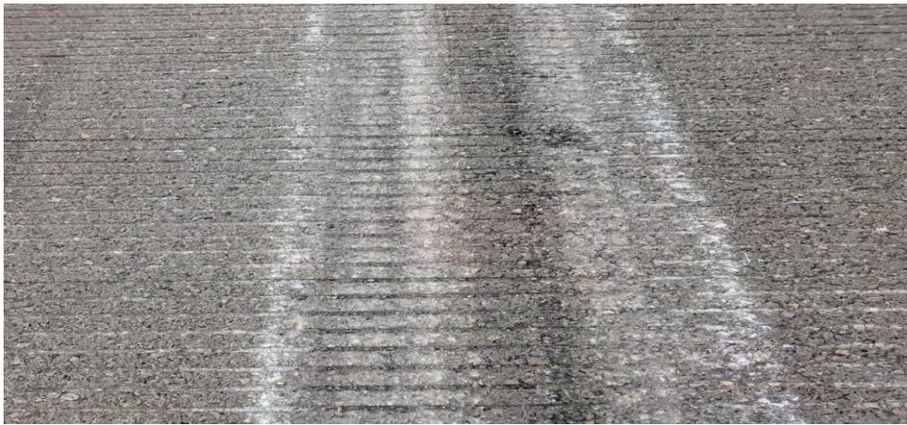
Figure 1: View of the skid mark on the runway created during the rollout phase by the left main gear wheel rims (#1 and #2)
