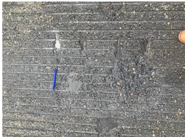
Figure 3: Crater created on the runway where the left main gear came to rest
